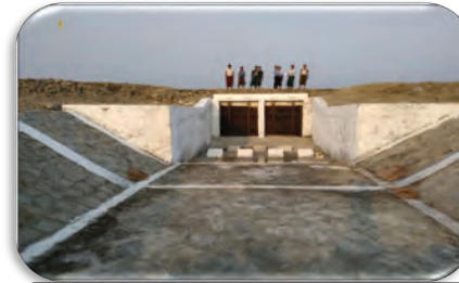
Construction of 2 Concrete Sluice Gates in Minbya Township
