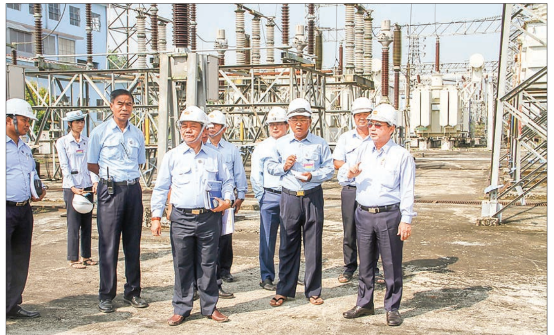
Deputy Minister U Khin Maung Win and officials inspect natural gas fired power station in Yangon. PHOTO: MNA
