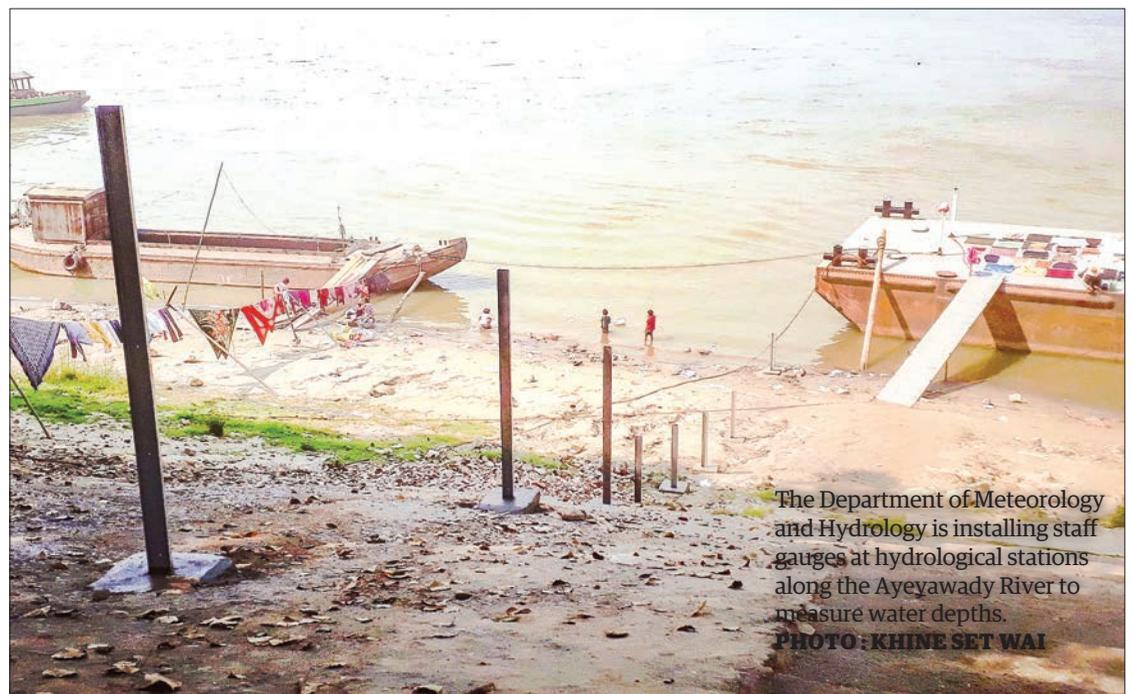
The Department of Meteorology and Hydrology is installing staff gauges at hydrological stations along the Ayeyawady River to measure water depths.
