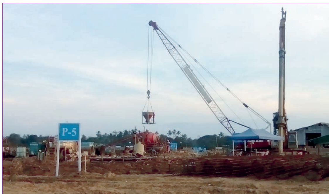
The Sittoung River crossing bridge (Oakphyat) is expected to be opened to traffic by 2021. PHOTO: SUPPLIED
