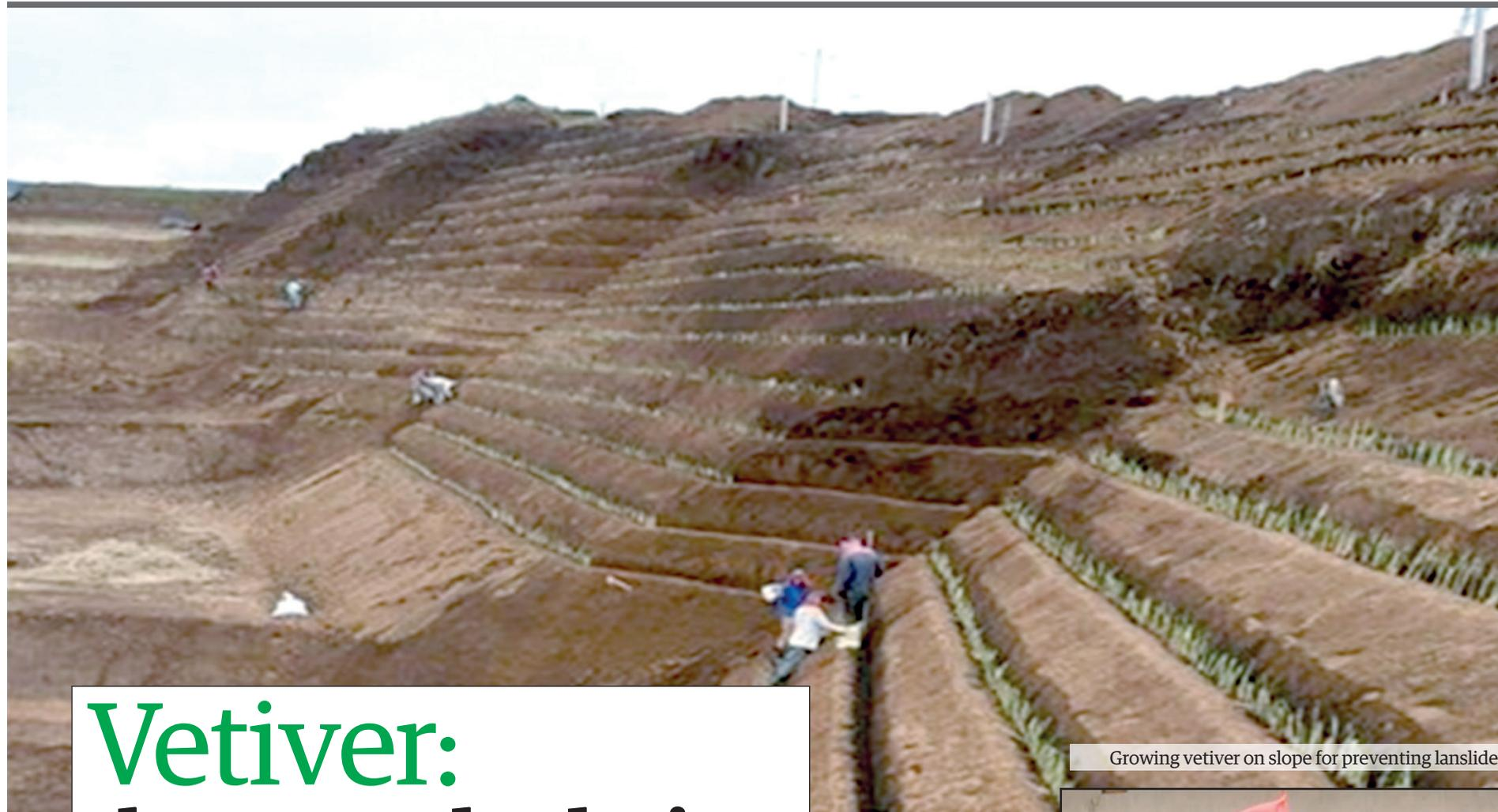
Growing vetiver on slope for preventing landslide
