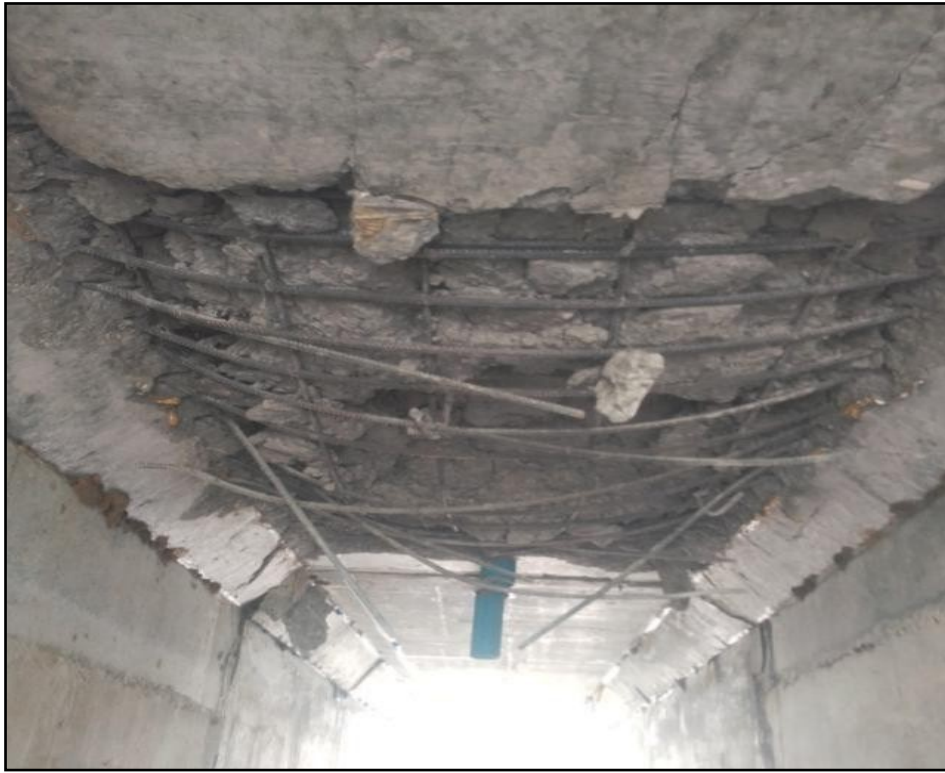
Damages of railway bridge between Painzalote and Tawwi Stations of Yangon-Mandalay Railroad in the aftermath of the mine attack of the terrorists
