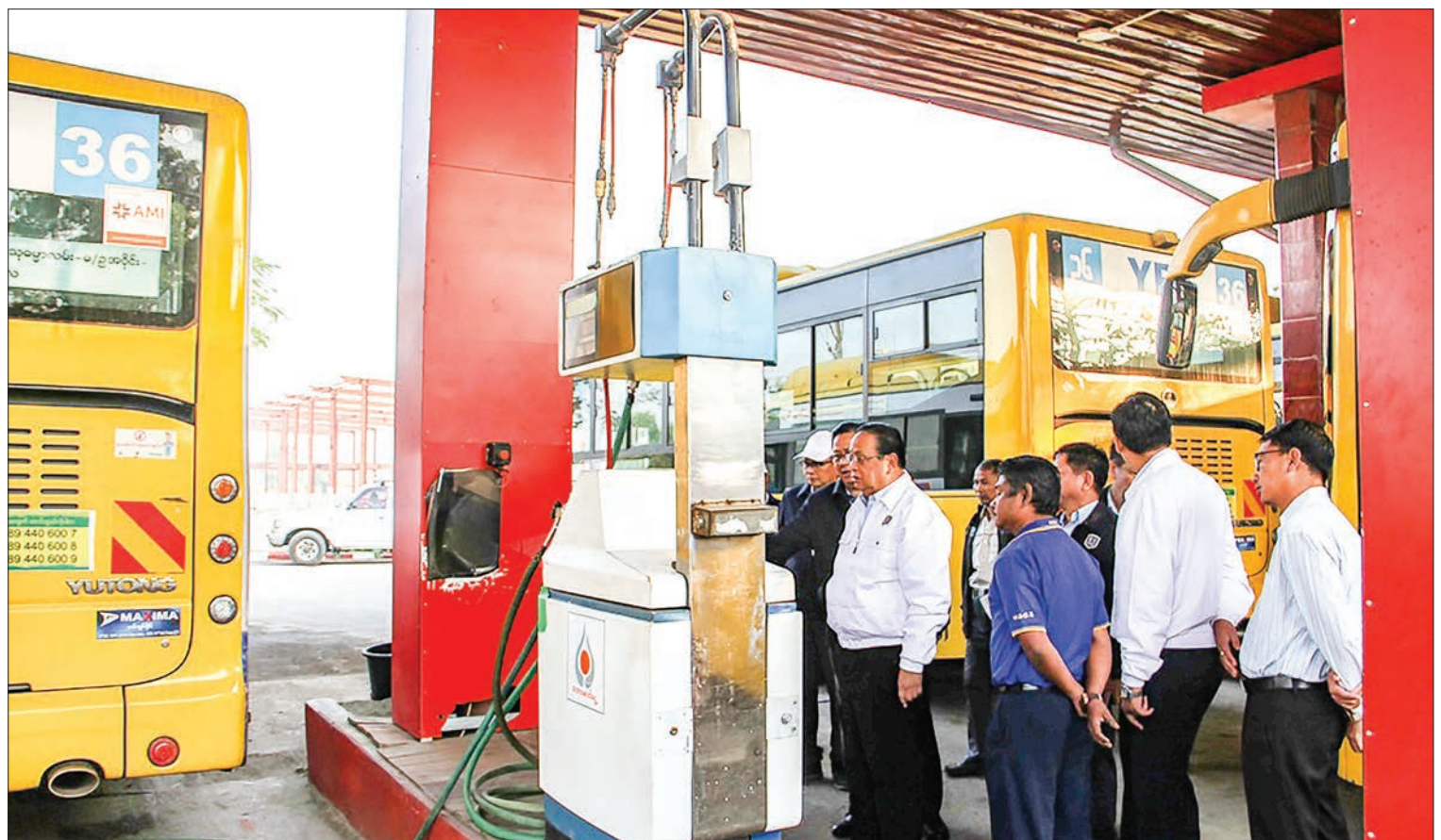
Union Minister U Win Khaing inspects CNG (compressed natural gas) refilling station in Yangon. PHOTO: MNA
